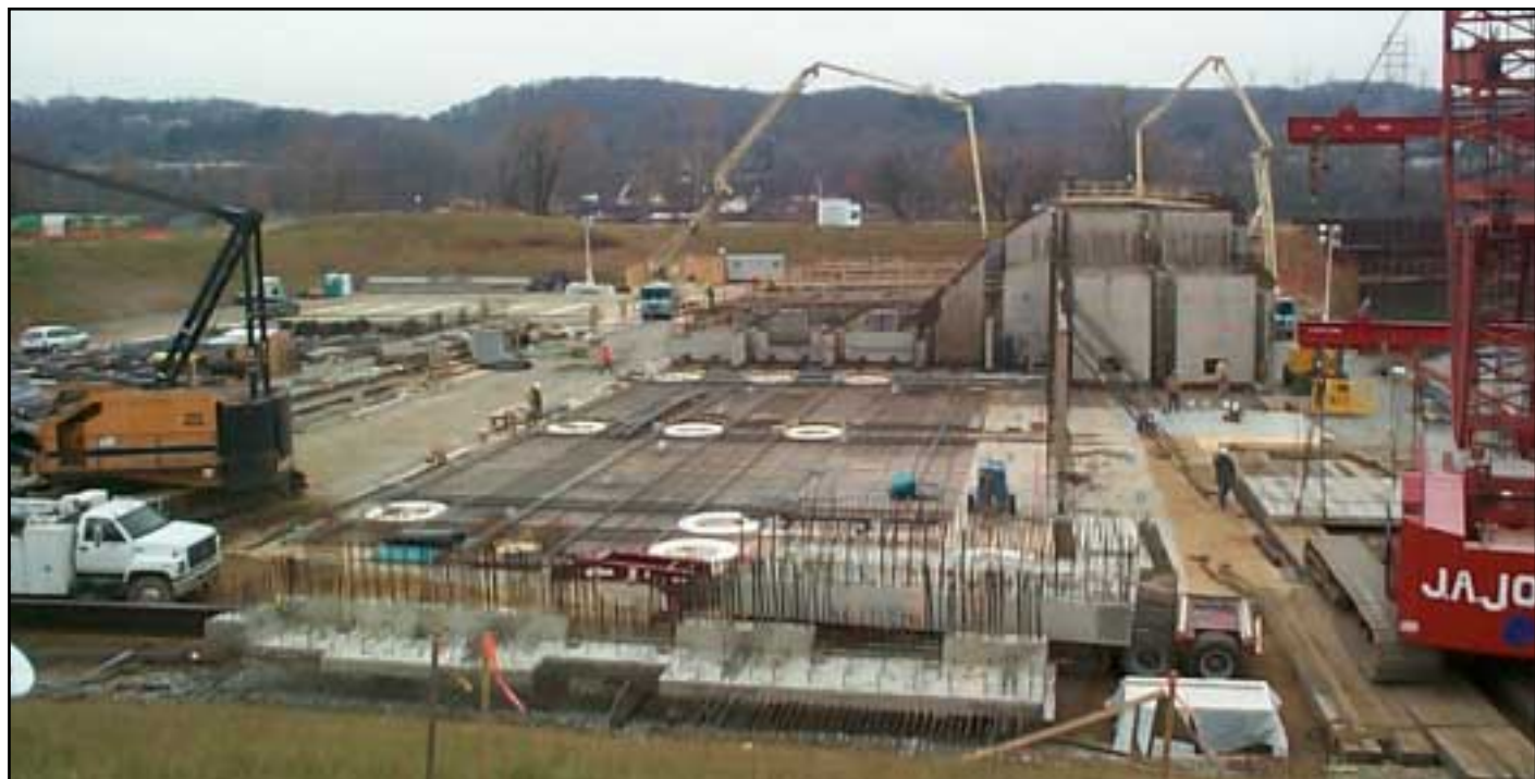
Dry dock construction
