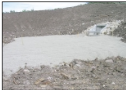
Jordanelle Ridge, Heber City, UT, Storm water rain basin after completion
