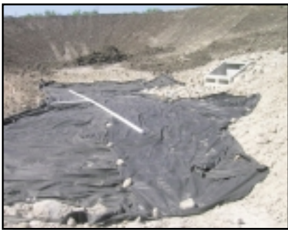
Jordanelle Ridge, Heber City, UT, Storm water rain basin under construction
